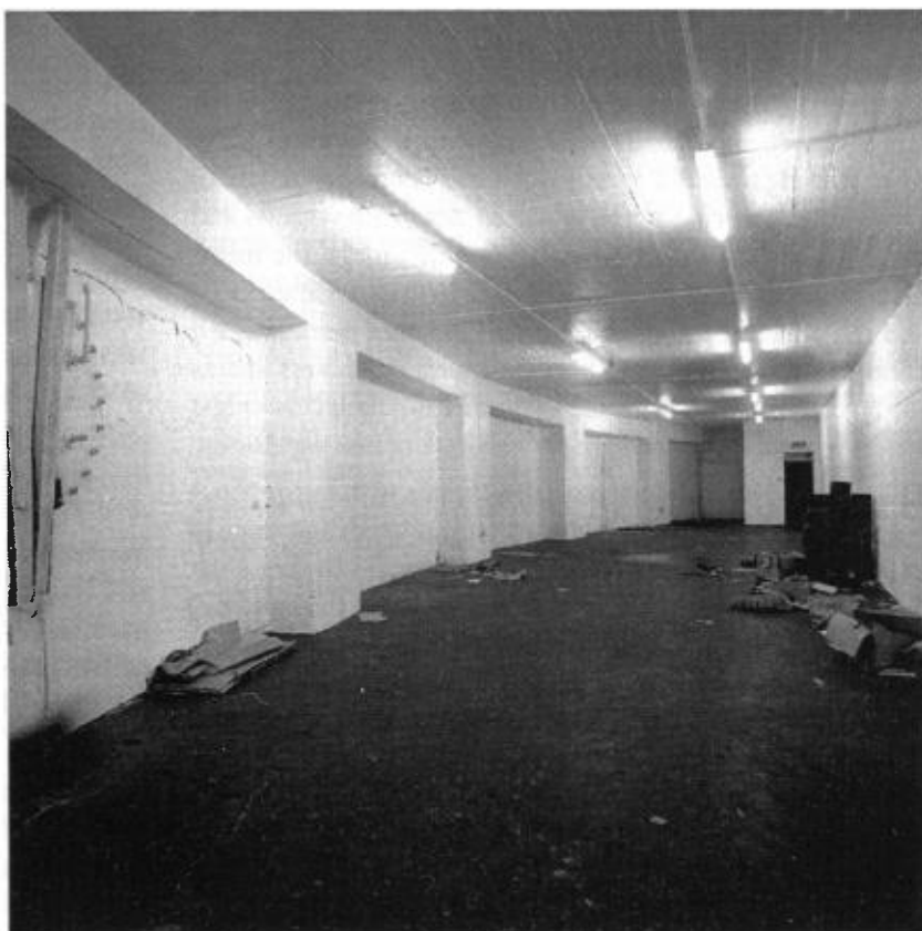
The curved internal wall clearly visible here
